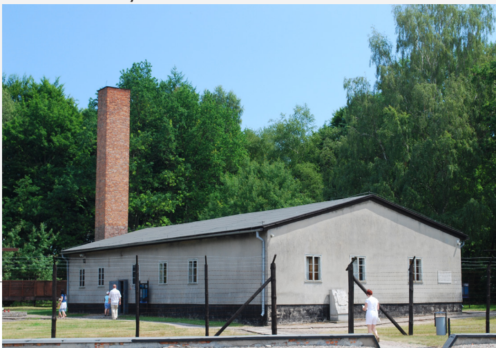
The building of the crematorium in the KL Stutthof camp.
